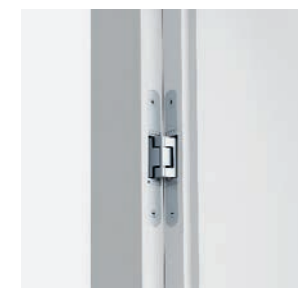
Door frame corner from hinges side
